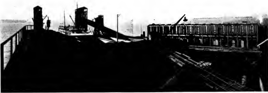
View on top of the Pacific Coast Coal Company's Seattle bunkers, showing towers and coal pockets.
